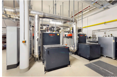
Fig. 6: Peak load boiler
